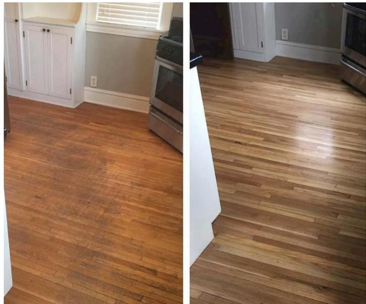
The transformation of an older Blackbutt floor after resanding and coating.
