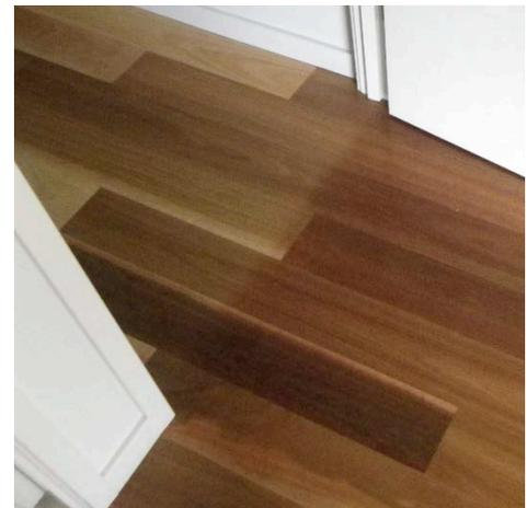
In the cupboard the floor is not exposed to as much light and the floor has not darkened.
