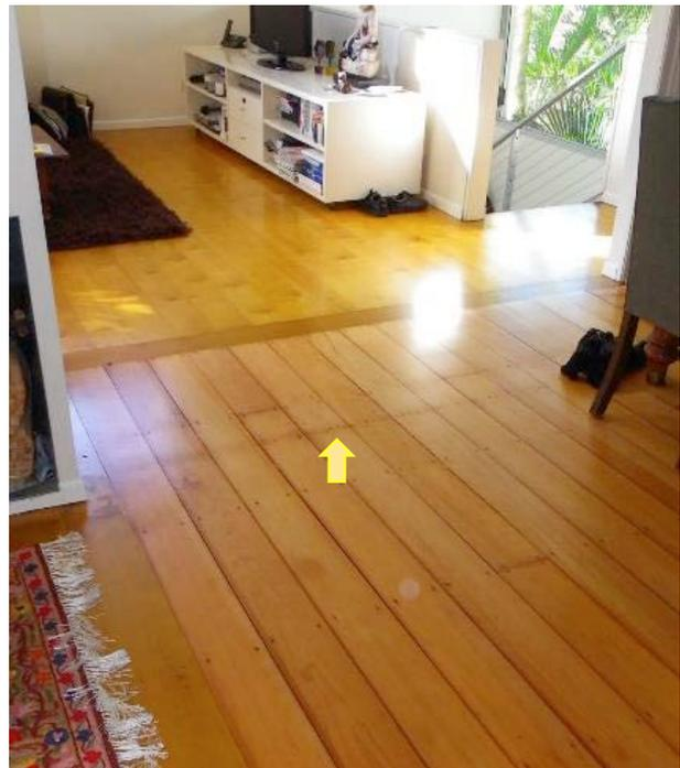
At the top of the photo the floor was not resanded and coated due to the architectural break. The resanded and coated flooring in the lower section of the photo had been tinted in an attempt to match. If it had not been tinted the boards would have looked 'white' in colour. Note also the arrow indicating a colour difference where a past internal wall had been present.
