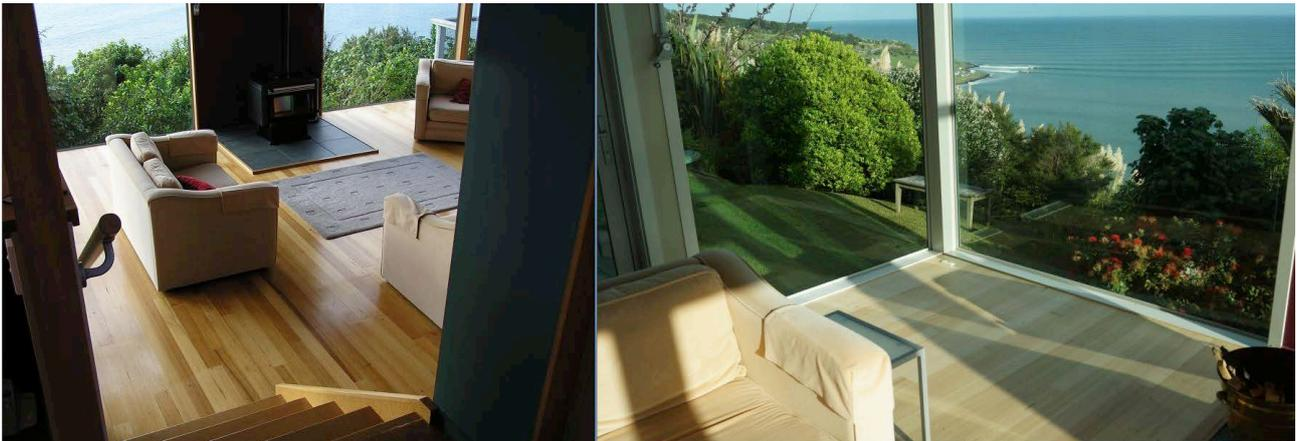
The photo on the left shows a floor with an aged oil-modified urethane and to the right a water based polyurethane on the same floor after about a year's service. It is important to note that the sealer used will also significantly influence colour as a floor ages.
